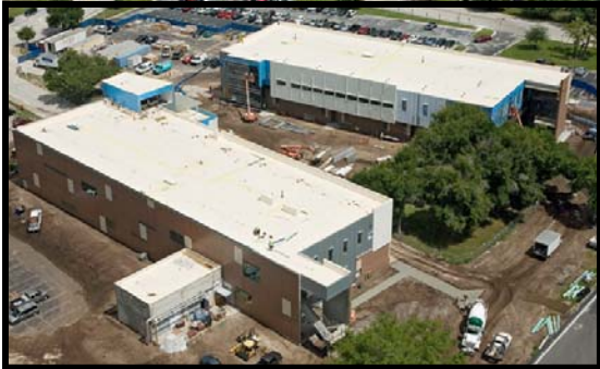
Performing Arts Complex Construction
